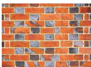
Diaper brickwork c.18 th Century.
