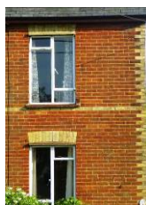
Contrasting quoin and string course c.1880.
