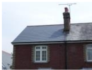
Slate Roof with Chimney Victorian
