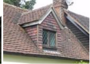
Roof with Dormer
