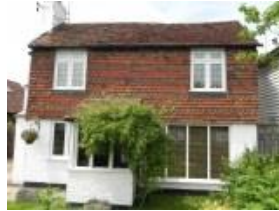
Cottage – render brick under plain roof tile
