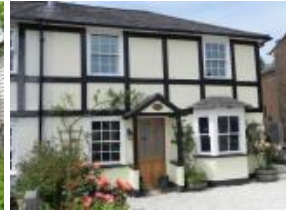
Timber panels inset
