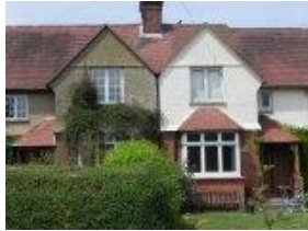
Gable into roof under render/pebbledash
