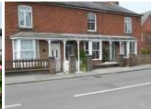
Canopy under brick elevation
